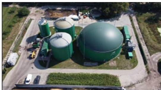
Figure 3: A Biogas Plant using Dynamic Technology (Source: Krzysztof et al. , 2025)
