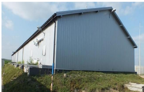
Figure 4: ProBioGas Plant Located in Międzyrzecz Podlaski (Source: Mahmoodi et al. , 2022)
