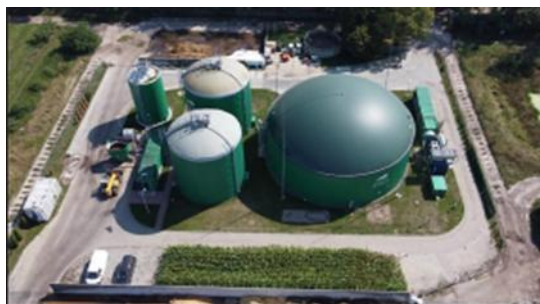
Figure 3: A Biogas Plant using Dynamic Technology (Source: Krzysztof et al. , 2025)
