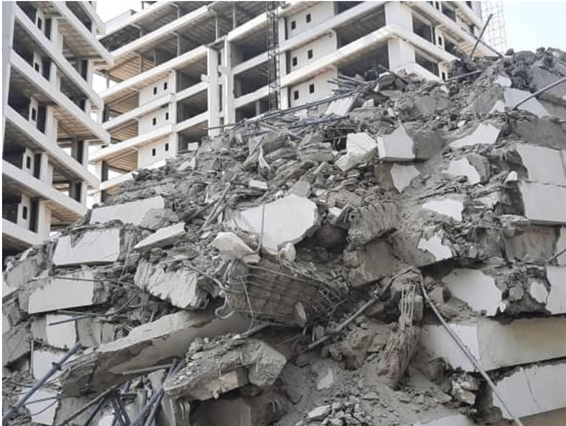
Plate 1: 21-storey luxury apartment building that collapsed during construction in Lagos (GCR, 2024)
