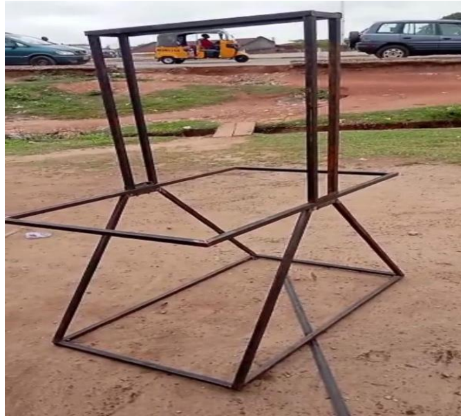
Plate 1: Constructed Structure of the Exterior and Interior Frames
