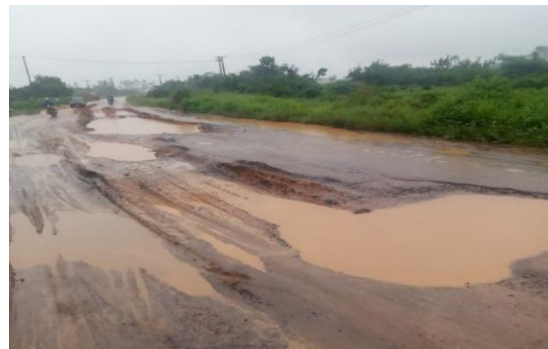
Plate 1: Photoshot of failed portions along New Eku Road, Sapele, Delta State, Nigeria
