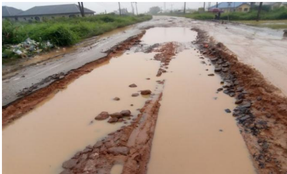
Plate 1: Photoshot of failed portions along New Eku Road, Sapele, Delta State, Nigeria
